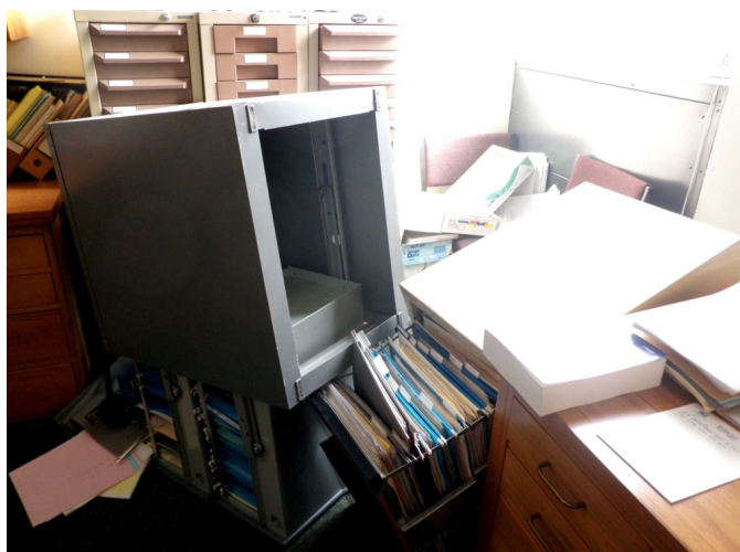
A consequence of stacked filing cabinets. Toppled cabinets would have presented significant threat to personnel if offices had been occupied during the earthquake.
